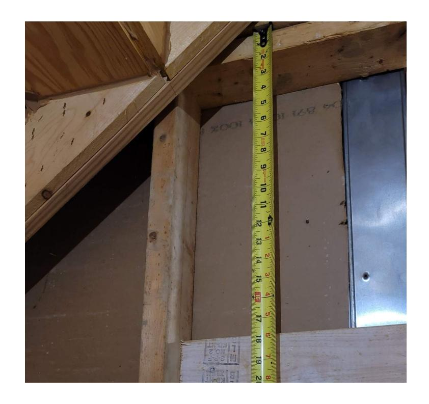
Using your measuring tape, measure the distance between the ceiling or top plate and the floor.
