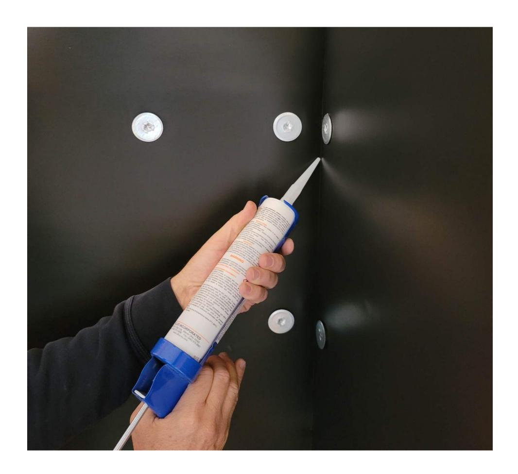
Caulk the perimeter seams with an acoustic sealant, such as OSI SC-175 Thermal & Acoustic Sealant, or Green Glue.
